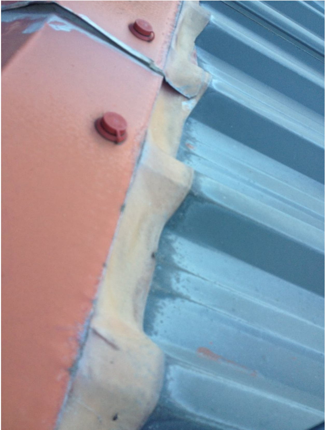
Caption lead in contact with coated or uncoated AZ will cause premature corrosion.
