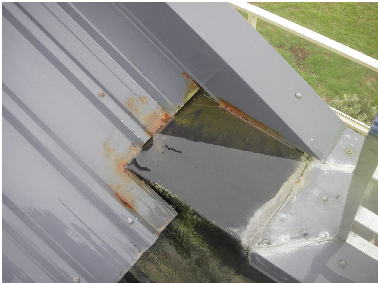
Butyl rubber in wet contact with coated aluminium and steel has been found to accelerate corrosion.
