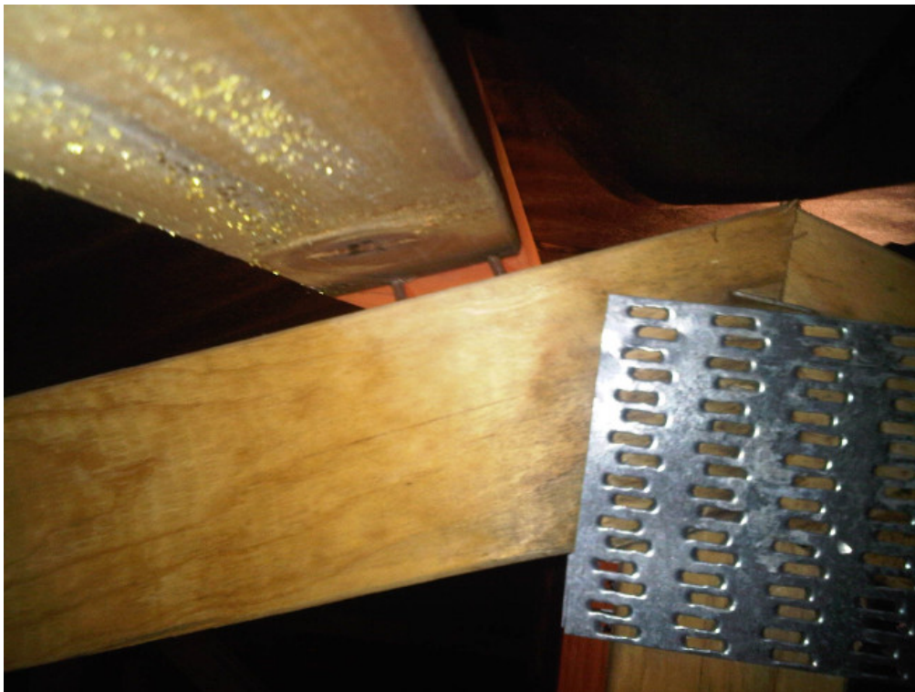
Poor purlin to rafter connection-tightness often causes noisy roofs.
