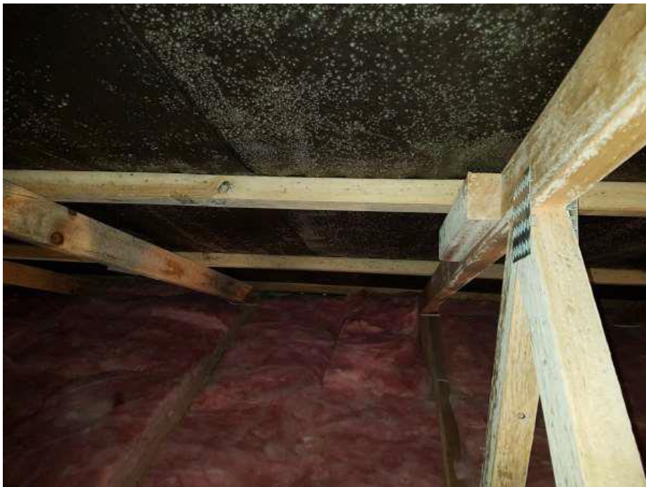
This building suffered mould damage to underlay and roof truss even before occupants moved in.
