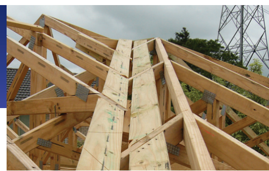
▲ Example of correct construction of valley boards
