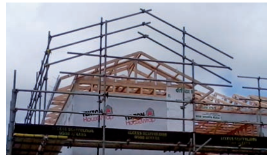
▲ Example of scaffold on gable ends
