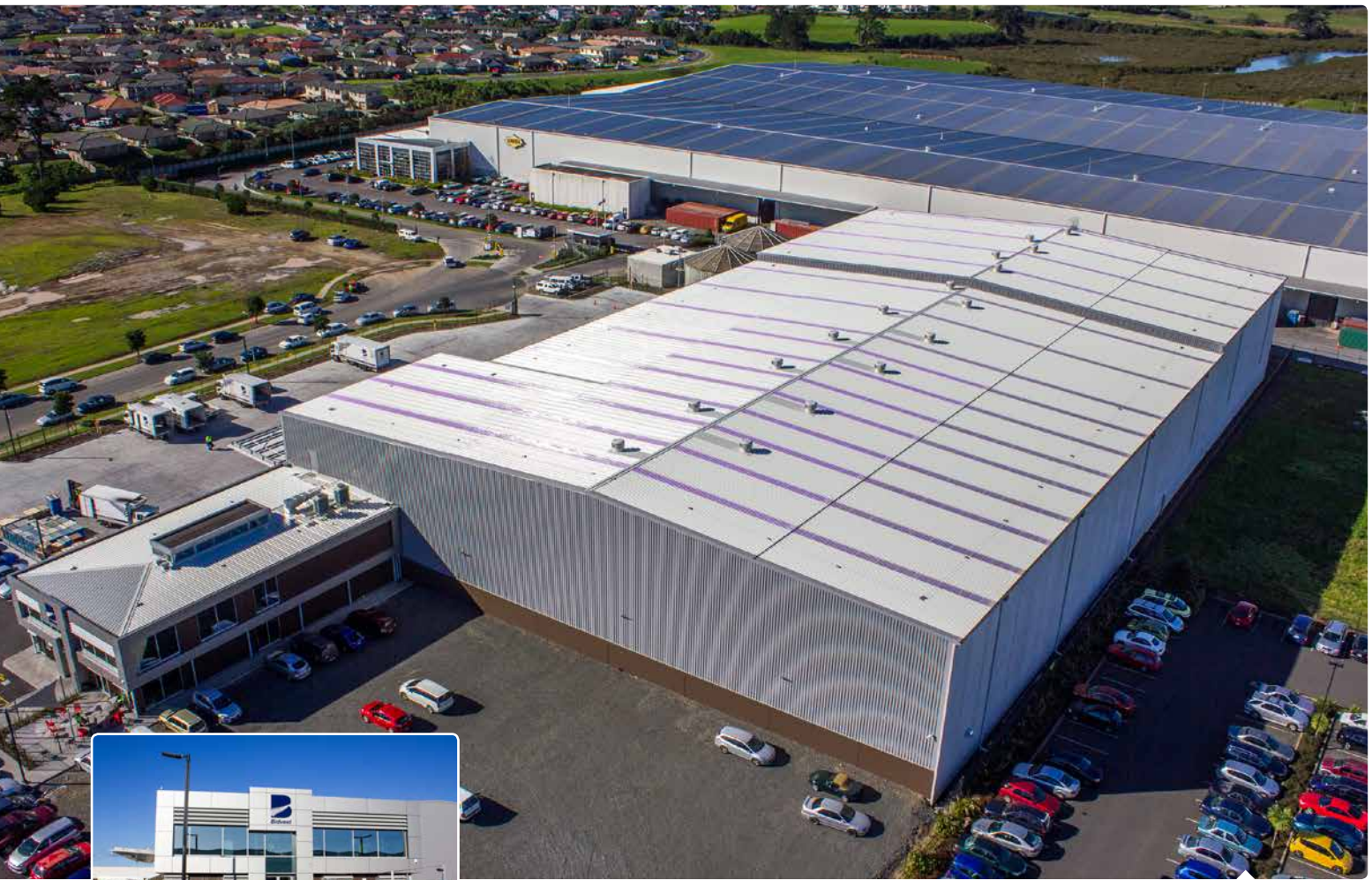
Bidvest NZ Ltd with Alsynite AITV 900 Ventilators
